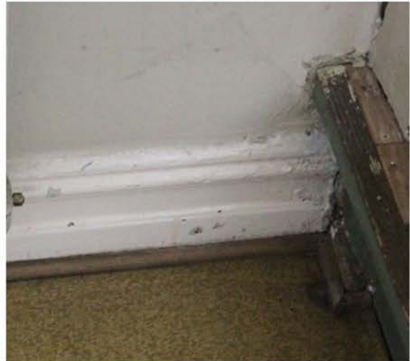
Sockel intill trappa – original.
